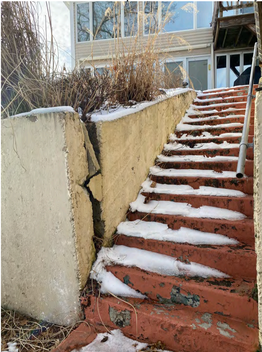
Picture Above: Existing Stairs
