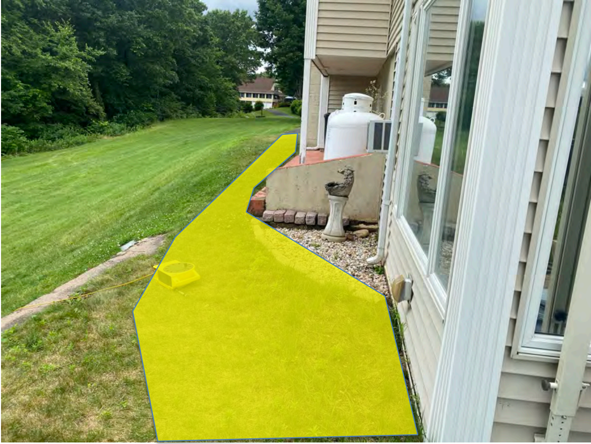
Picture Above: Area for new paver walkway from existing patio to driveway, approximately 55' long x 42" wide. Existing pavers on site to be reused for this new walkway.
