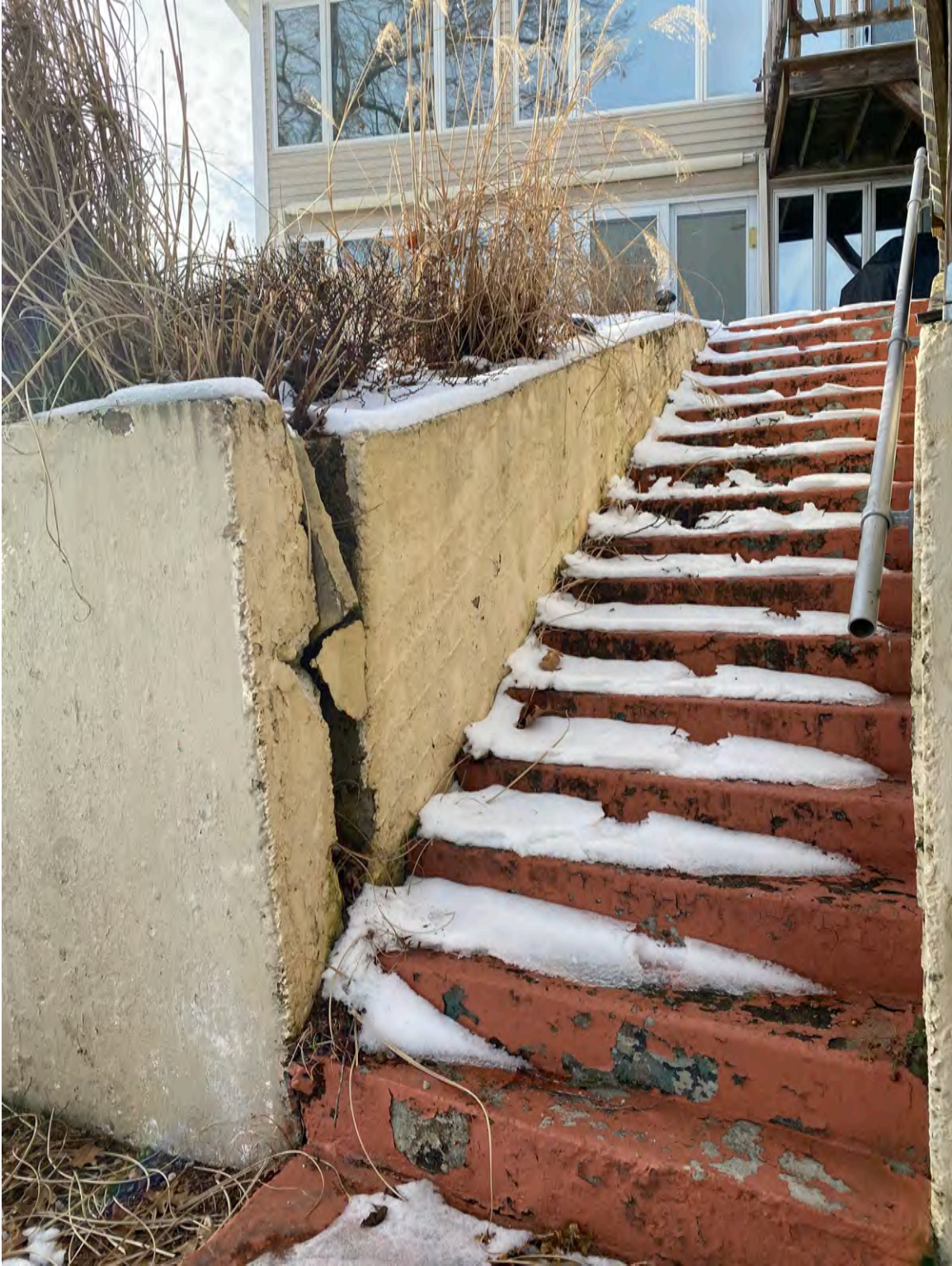
Picture Above: Existing concrete stairs to be removed
